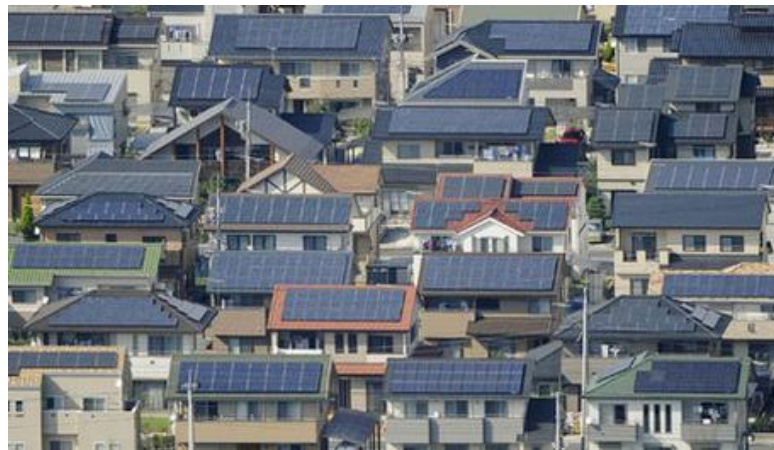
Solar PV on homes in Yokohama City
